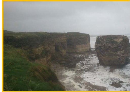
Rockfall, caves and extensive fissuring of cliff face
