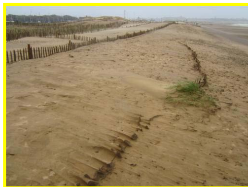
Dune fencing well buried in places with some signs of new vegetation growth.
