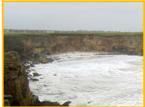
Historic collapse of cliff at centre of bay has not worsened.
