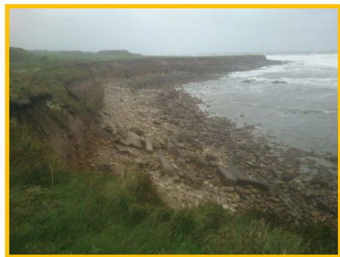
Concrete blocks dumped to protect cliff toe.
