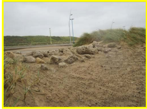
Placement of cobbles at the blowouts in the dune crest
