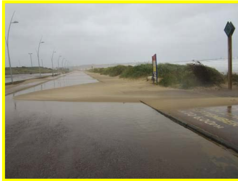
Windblown sand on the promenade at the access ramp and blowouts.
