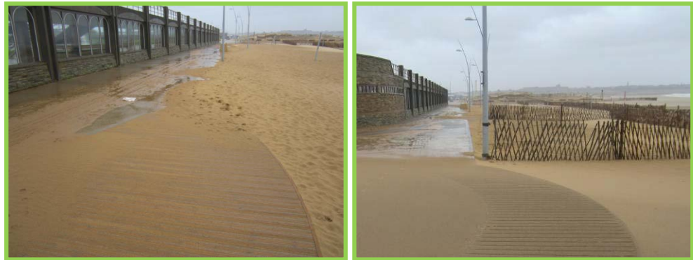
Windblown sand on the new promenade at the Amphitheatre. Dune fencing along the back of beach at the Amphitheatre
