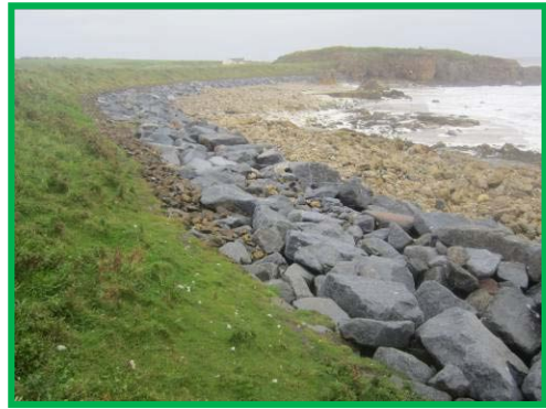
Rock armour well interlocked with no signs of settlement or movement.
