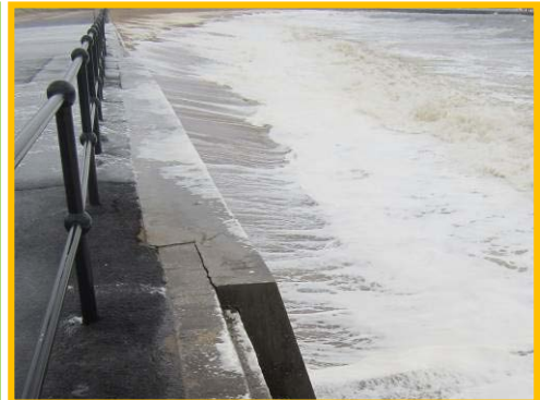
Gaps behind concrete facing at south end.
