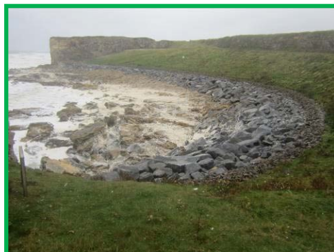
Rock revetment in Southern Bay in good condition.
