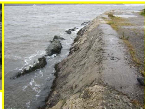
Concrete repair to face of revetment at north end.
