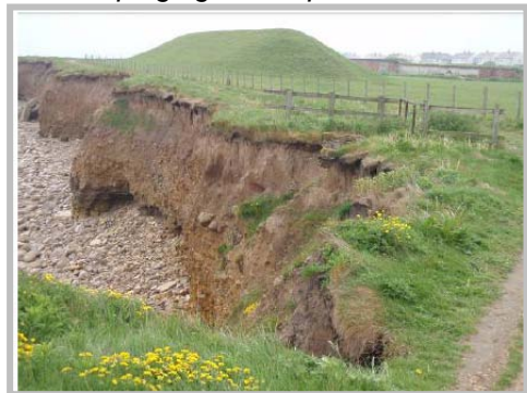
Photo from 2010 inspection report
