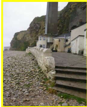
Masonry wall at Marsden Grotto protected by cobble berm.
