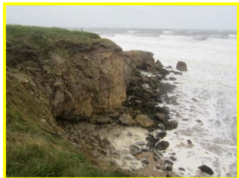
Rockfalls along the south face of Trow Point.
