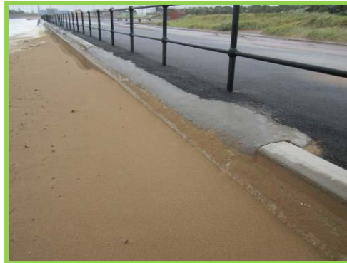
Repairs to missing coping stones remains in good condition.
