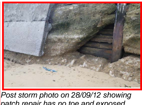
Gaps behind concrete facing at south end.
