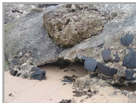
Photo of same location as above taken from 2010 inspection report
