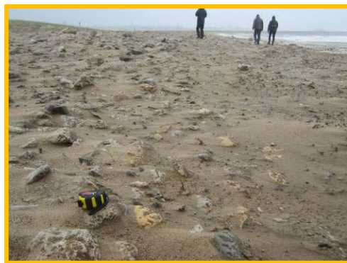
Wide cobble berm across beach at South Groyne.
